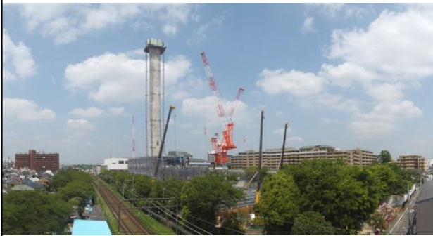
Suginami Incineration Plant (under construction)
