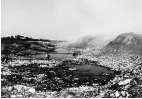
1910s Open-air incineration
