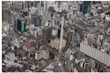
Shibuya Incineration Plant
