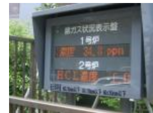
Incineration plants display gas status on a display in real time (Setagaya Incineration Plant)
