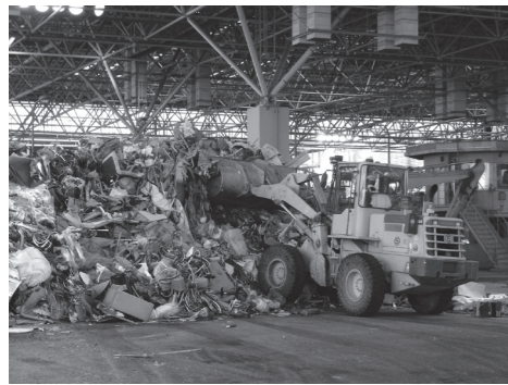
Receiving yard at a Large-sized Waste Pulverization Processing Facility
