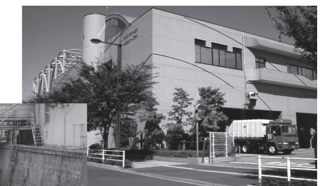
Land Transfer Station (Shinjuku Transfer and Resources Center, Shinjuku City)
