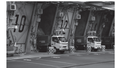
Waste unloading (a platform at Adachi Incineration Plant)
