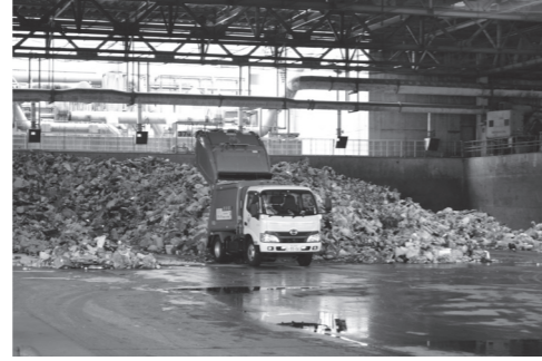
Incombustible waste is unloaded at a receiving yard
